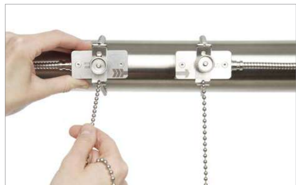
Transducers mounted using chains and clips
